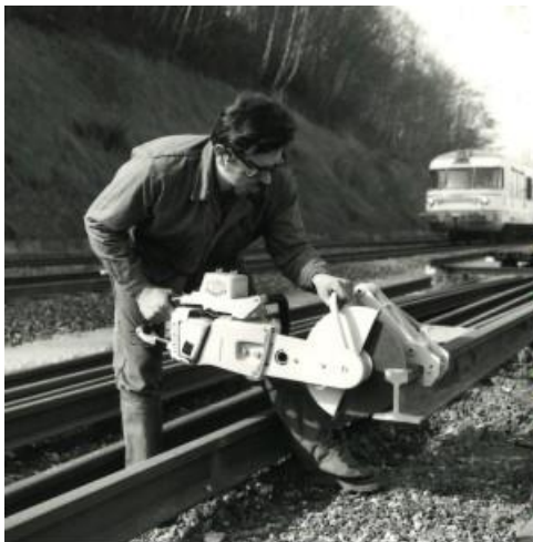
Geismar MTX rail cutter
